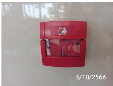
Fire Alarm Manual Station
