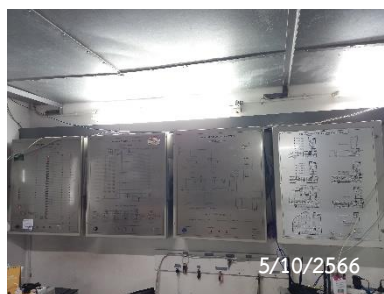
Graphic Annunciator Fire Alarm System
